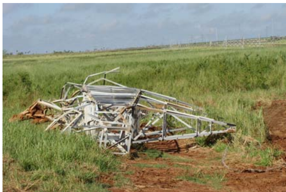
The wreckage of a downed electrical tower.
