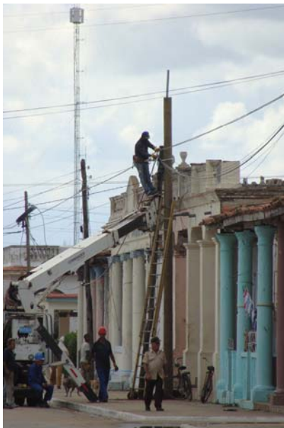
Relief and repair crews were active in Los Palacios.
